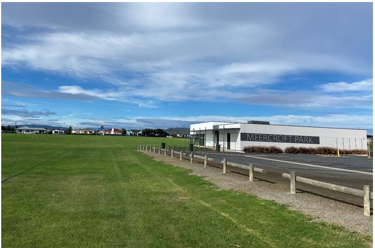
Meercroft Park (Source: Photo by Don Rockliff, GHD)
